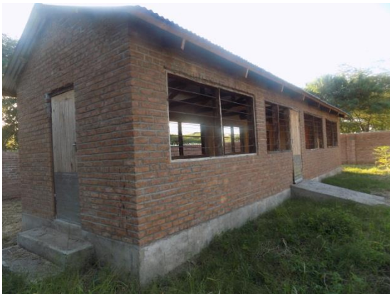
Figure 4 Deep litter house
